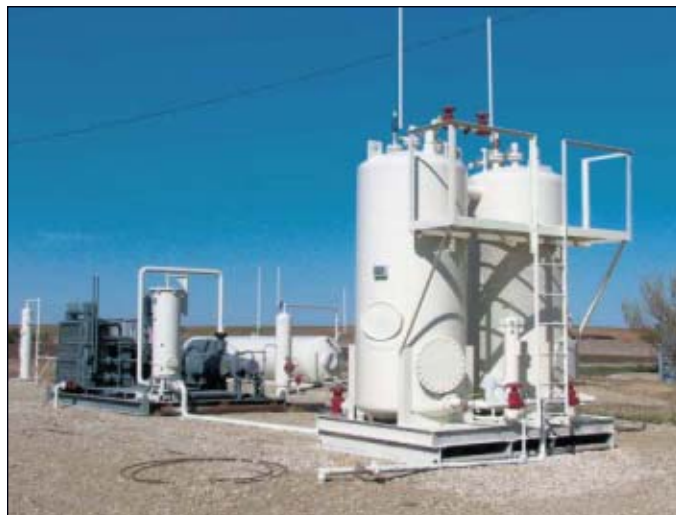
Nitrogen rejection alternatives in the Midcontinent range from the IACX Energy mobile unit at Otis, Kan., (top left) that uses nitrogen sponge technology to the smaller American Energies Corp. plant at Elmdale, Kan., developed with aid of a grant from the Stripper Well Consortium, 2 that uses the pressure swing adsorption method (top right) to BP American Production Co.'s cryogenic gas processing plant at Ulysses, Kan. (below). BP photo by John Charlton (Fig. 8).
