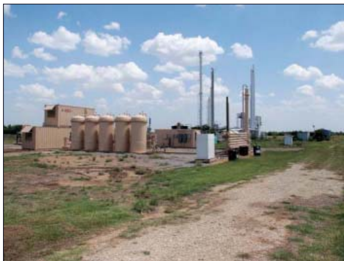
Nitrogen rejection alternatives in the Midcontinent range from the IACX Energy mobile unit at Otis, Kan., (top left) that uses nitrogen sponge technology to the smaller American Energies Corp. plant at Elmdale, Kan., developed with aid of a grant from the Stripper Well Consortium, 2 that uses the pressure swing adsorption method (top right) to BP American Production Co.'s cryogenic gas processing plant at Ulysses, Kan. (below). BP photo by John Charlton (Fig. 8).
